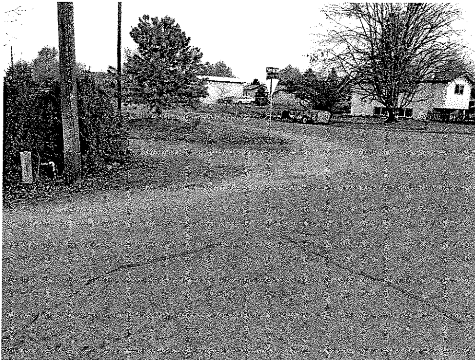
Figure 5 – Looking Southeast at the Binford Drive & Friends Road Intersection
