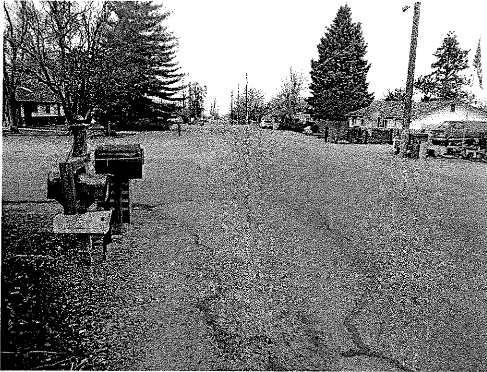
Figure 4 – Looking North from Southwest Corner of Butler Lane & Friends Road Intersection
