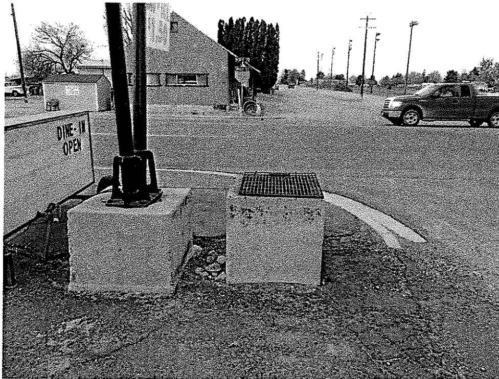
Figure 3 – Looking North from Southwest Corner of SH-19 & Friends Road Intersection
